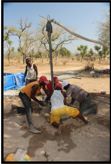
The well going in at Djibir
